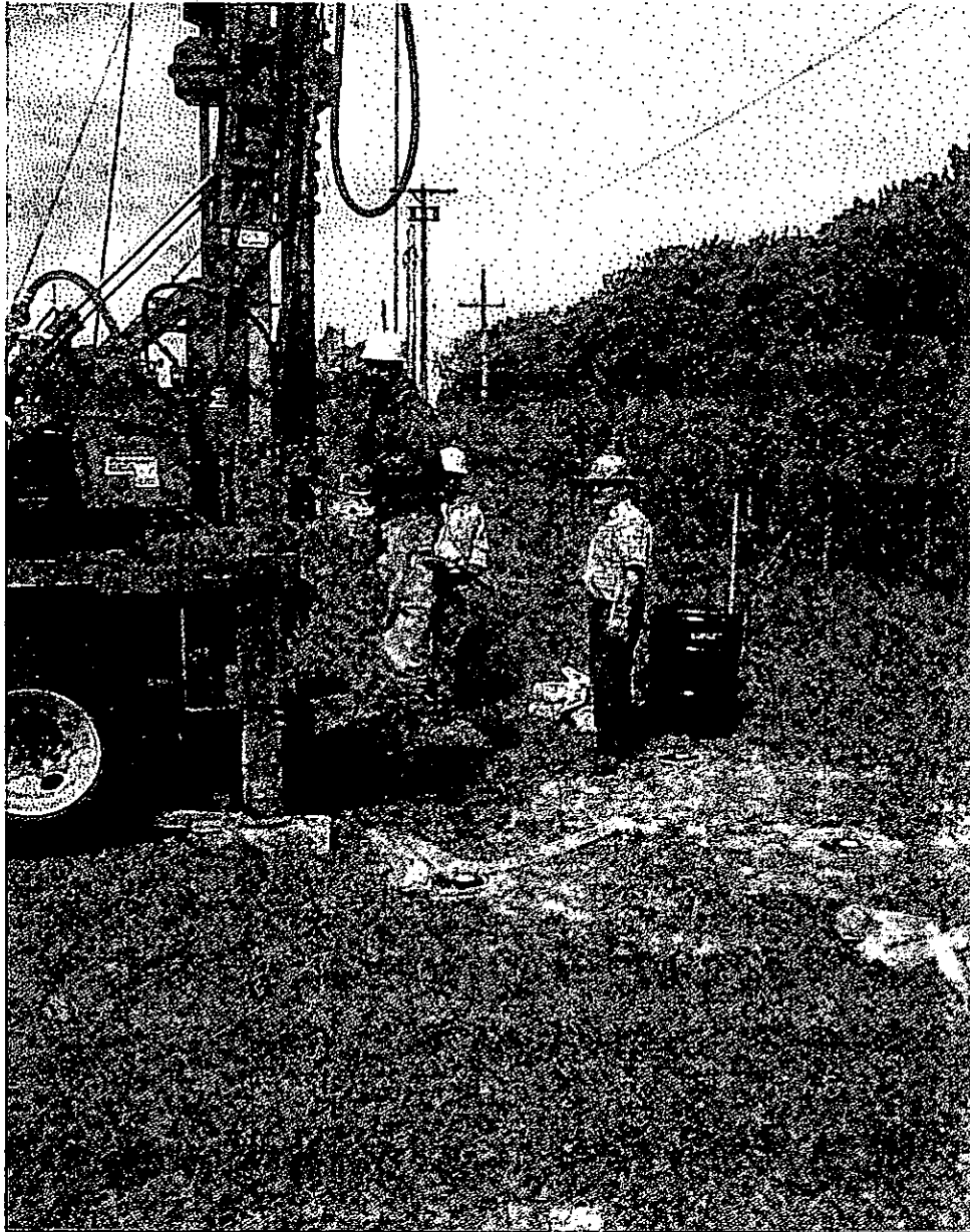
Installation of MW-5 through MW-8
